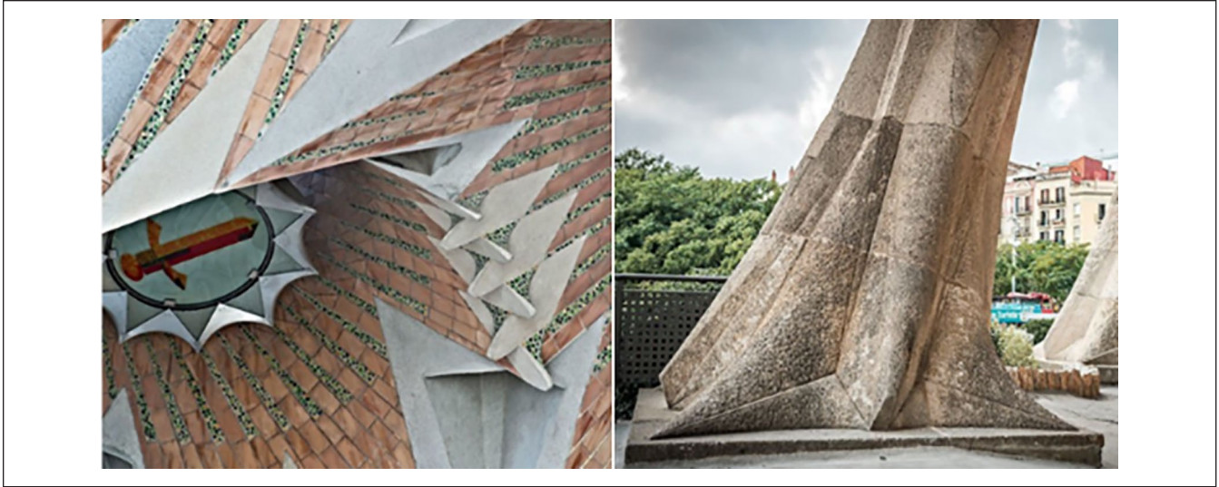
Figure 8. Hyperbolic surfaces and parabolic pillars of The Sagrada Familia (URL-4).
