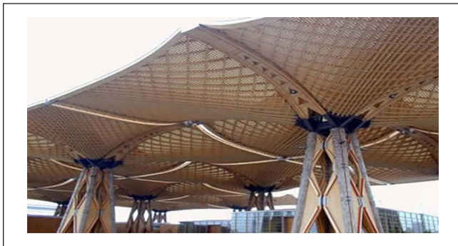
Figure 13. Tree-like structures designed for Expo 2000 (URL-9).
